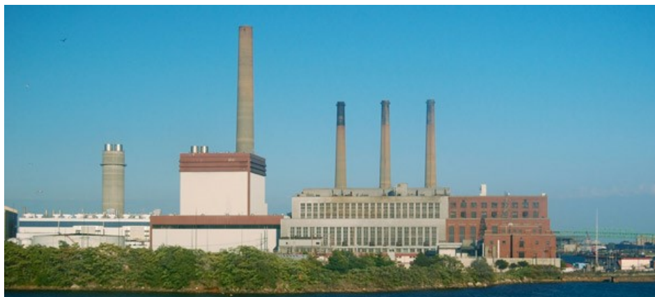
Mystic Generating Station
