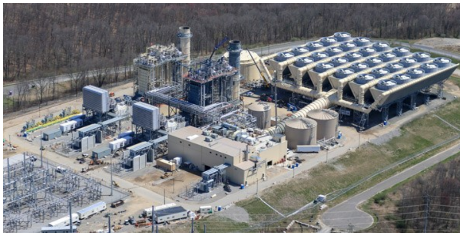
CPV Towantic Energy Center in early May, with construction nearly complete. | Competitive Power Ventures
